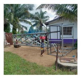
Water, a mainstay of life! **We have started the "Water Tower Project".** A second contractor has been chosen with a better price and using galvanized and PVC pipes and a 1000 gallon Poly Tank to be mounted on the 18ft high water tower. It also includes a submersible pump. The price is \$3000 USA.
